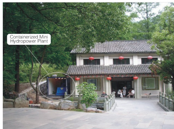
● 新老电站厂房对比 / Compared with the old powerhouse
