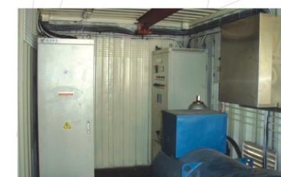
出线模块 —— 机组出线开关柜(图片左侧) Outlet module —— Circuit breaker panel (the left panel in the picture)
