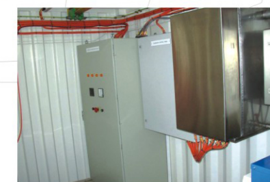
控制模块 —— 机组控制测量保护柜 Control module —— Control, measuring and protecting panel
